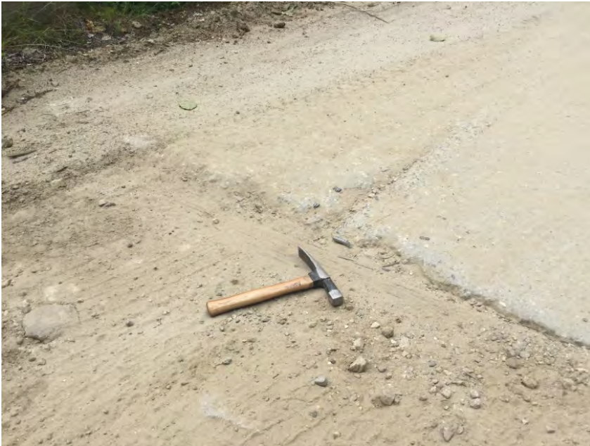
Wear of Girder in Wheel Track at Left Abutment
