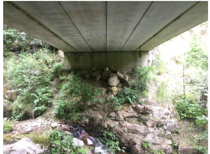
Right Bank Abutment
