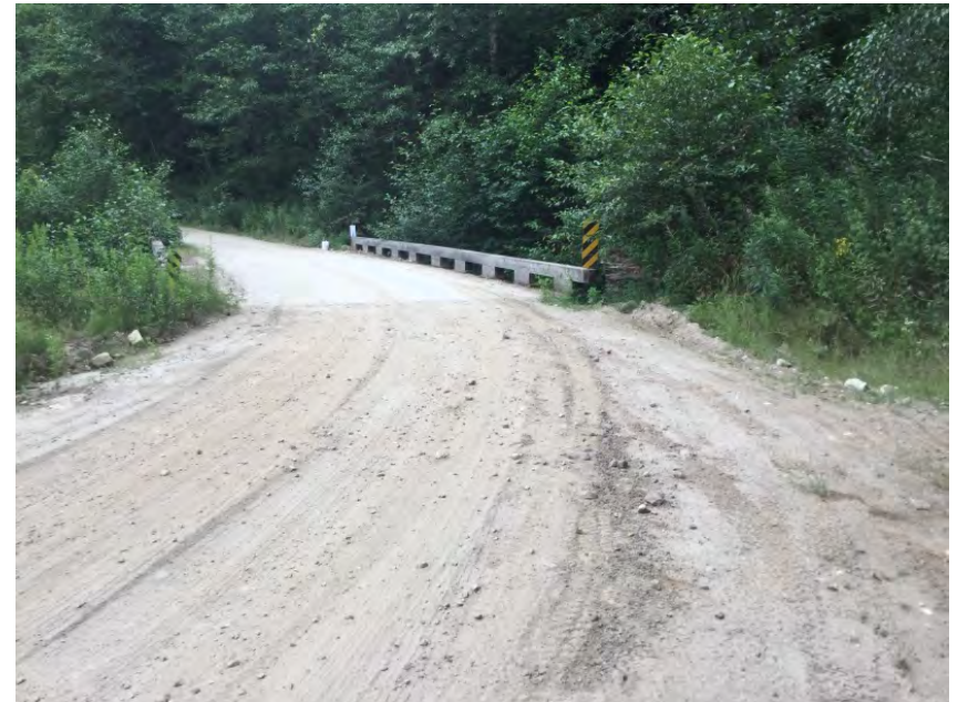
Left Approach Facing Bridge
