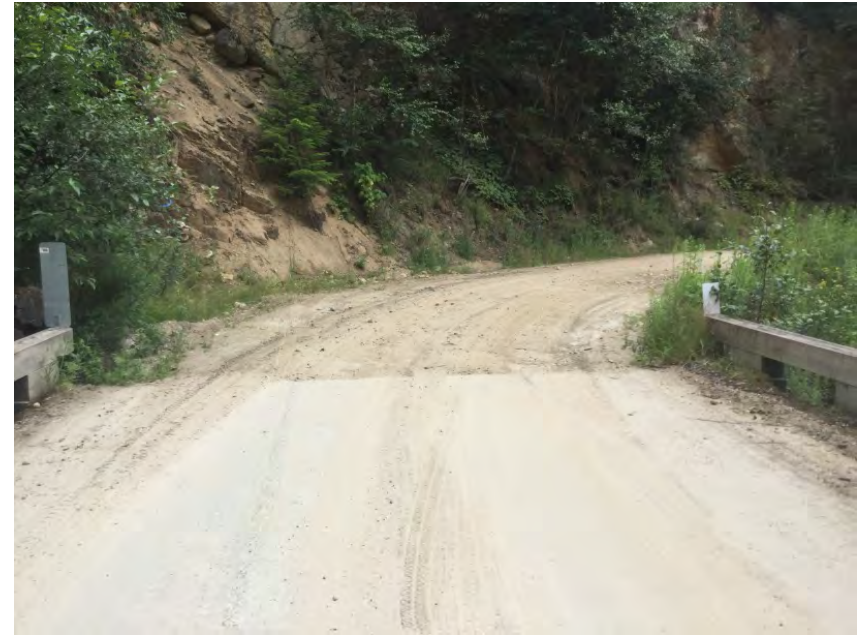
Left Approach Facing Away From Bridge
