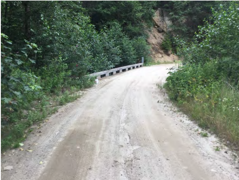
Right Approach Facing Bridge
