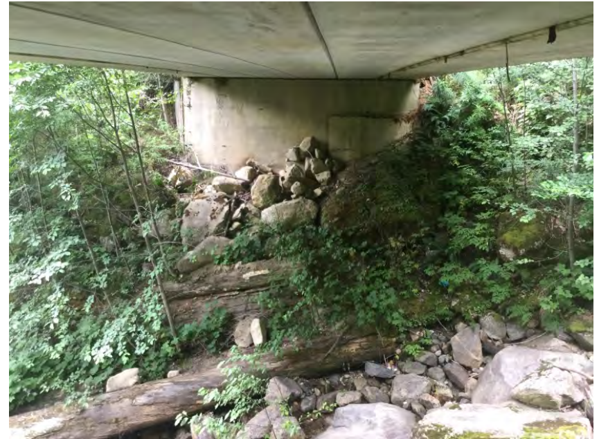
Right Bank Abutment
