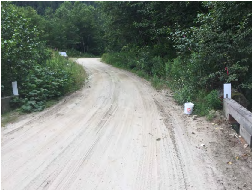
Right Approach Facing Away From Bridge
